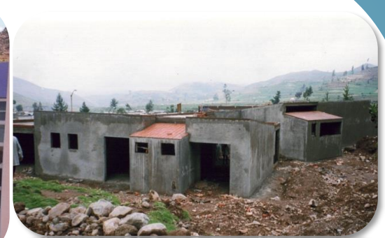
Bau Spital Chuquibamba
